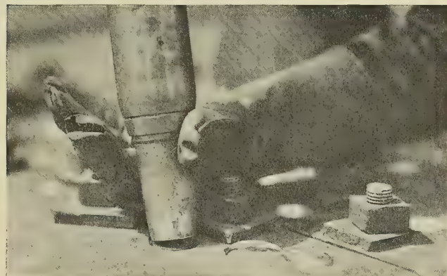
Fig. 20.—Calking Finished Rivet While Still Hot
